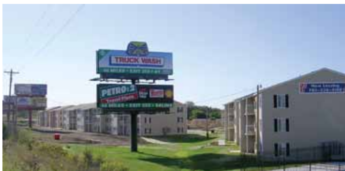
The Geary Estates apartments, located off I-70 and exit 301, have expanded adding new members to Flint Hills RECA.
